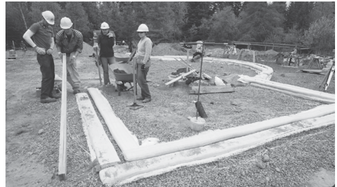
Earthbag foundation. (DAVID ELFSTROM)
